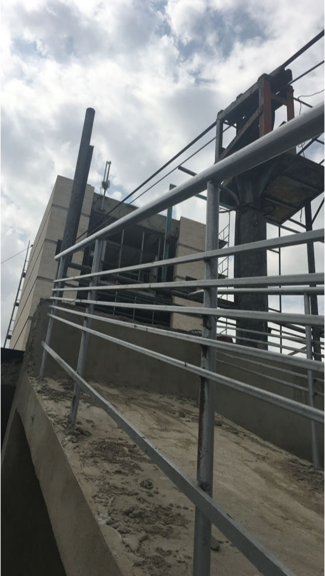
View of the of the upper station building [Image: authors]
