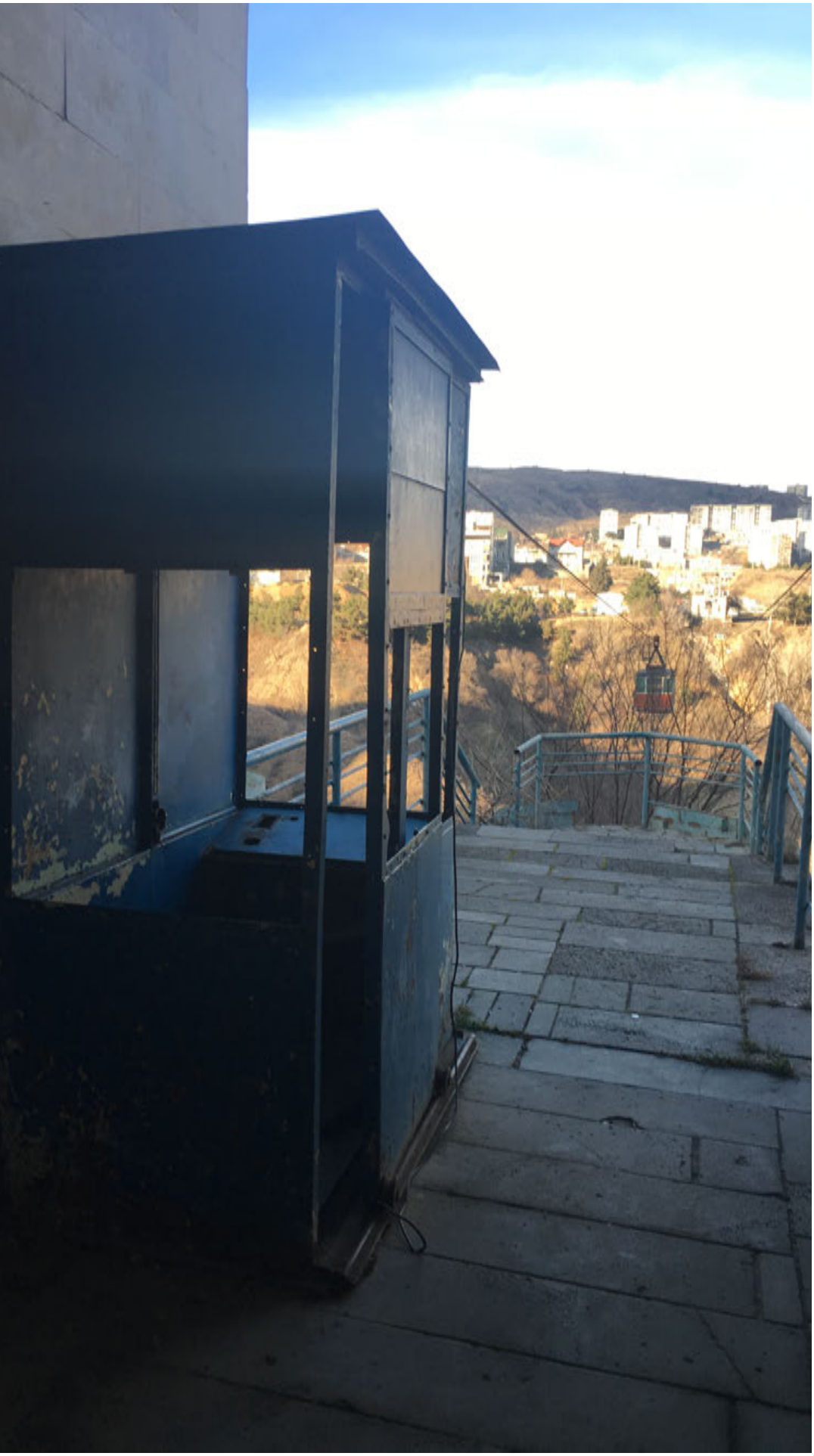
View of the of the station building interior [Image: authors]
