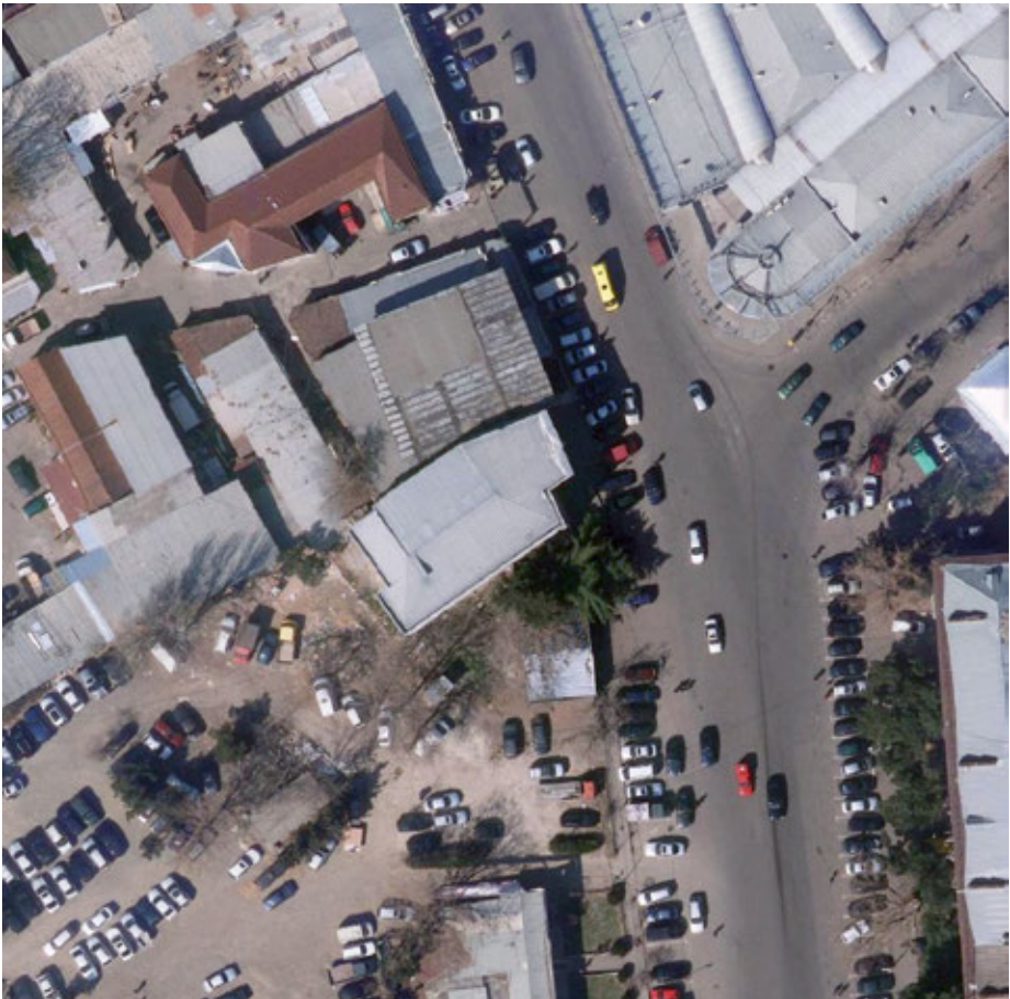
Aerial view of the former station building inside Iliava market
