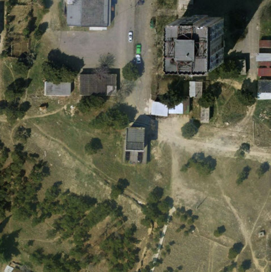
Aerial view of the upper station building near Vazisubani
