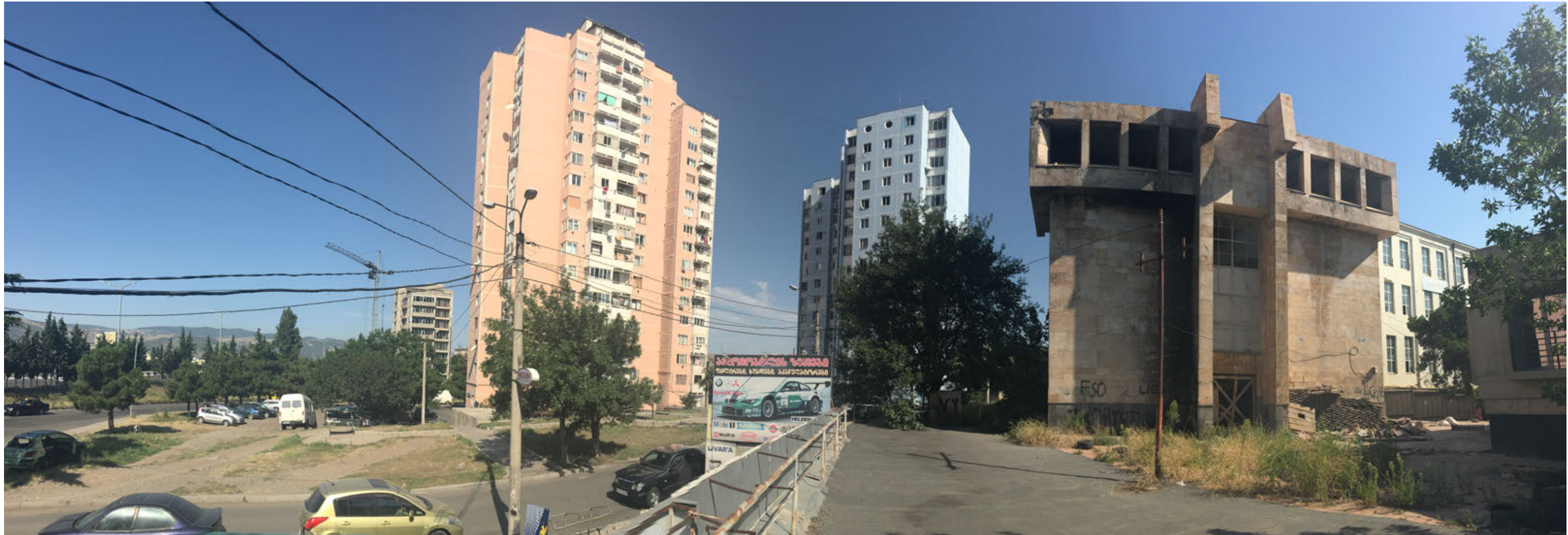
View of the exterior of the lower station building [Image: authors]
