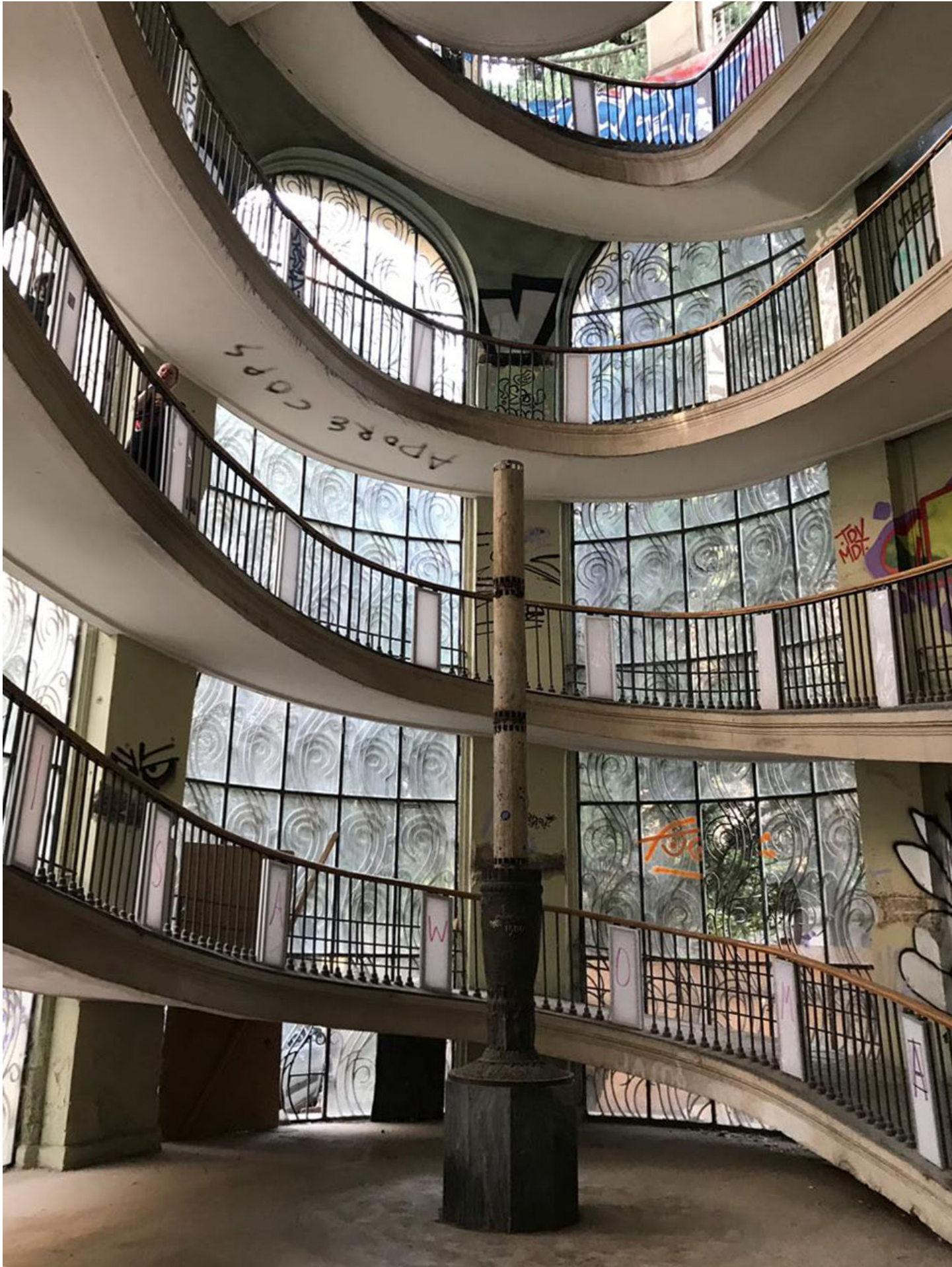
View of the interior of the lower station building [Image: authors]
