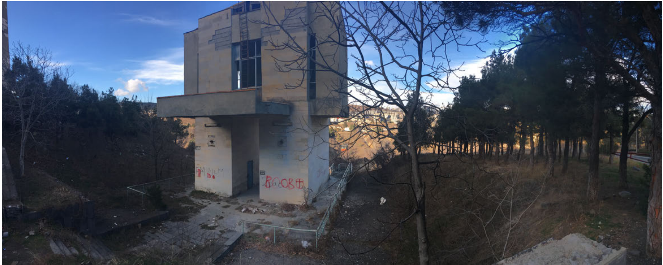
View of the of the dormitory-side station building, prior to reconstruction [Image: authors]
