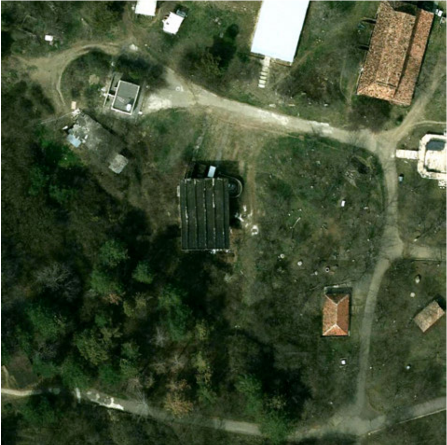
Aerial view of the lower station building
