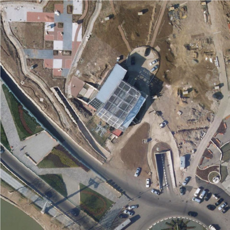
Aerial view of the lower station building in Rike Park, under construction
