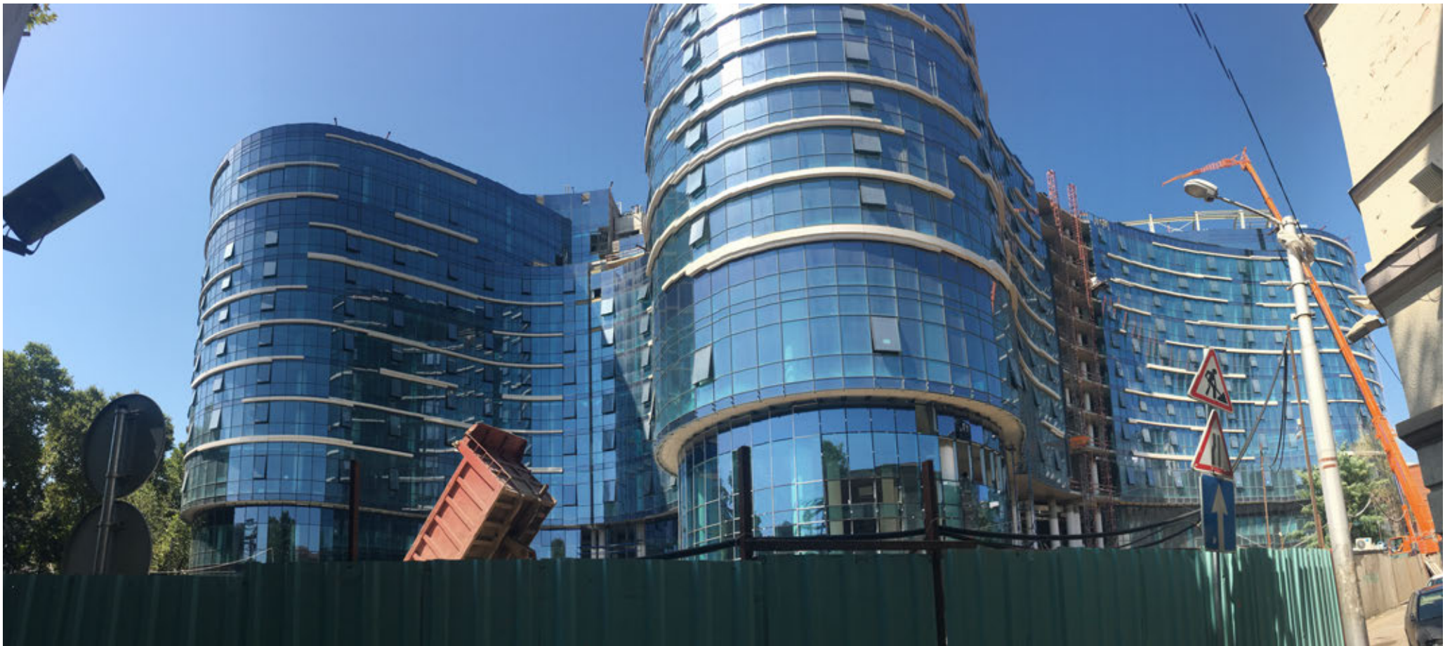
View of the Liberty Square building of Panorama Tbilisi project, under construction 2019 [Image: authors]
