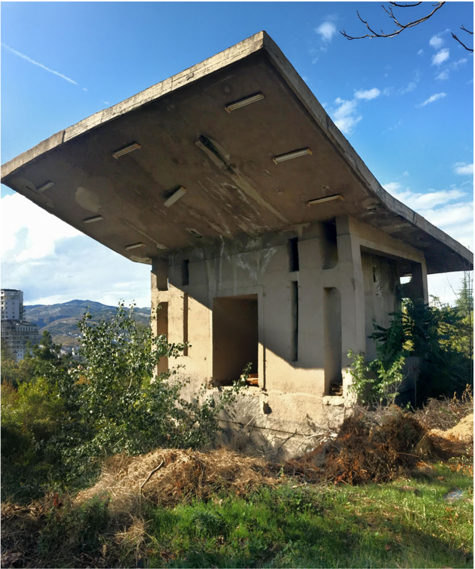
View of the back exterior of the lower station building [Image: authors]
