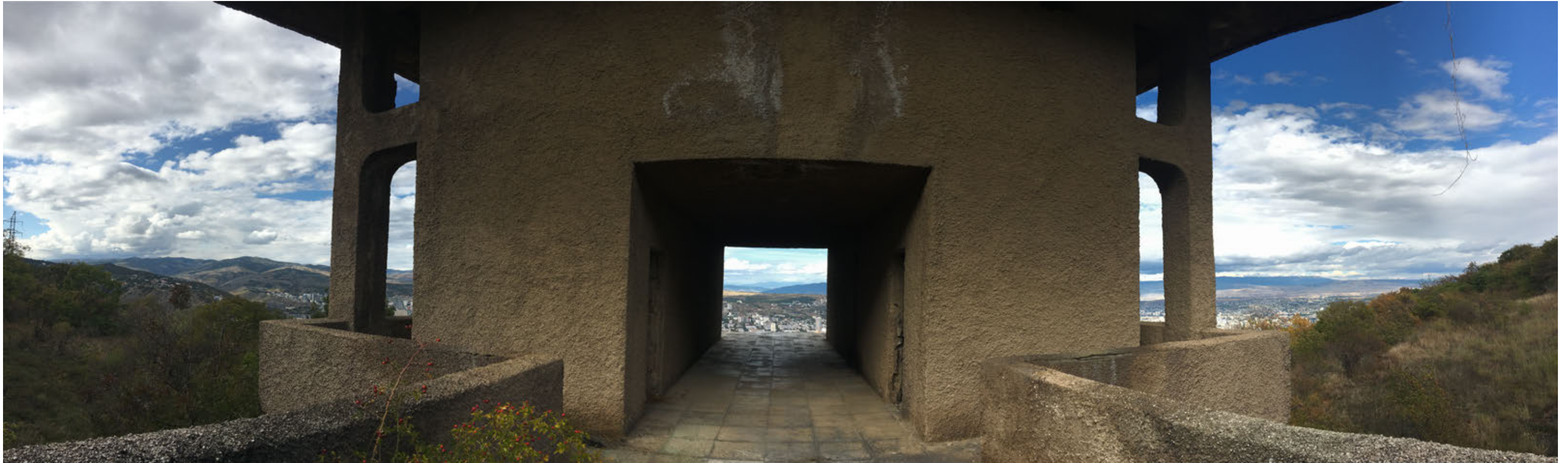
Panoramic view of the upper station building entrance [Image: authors]
