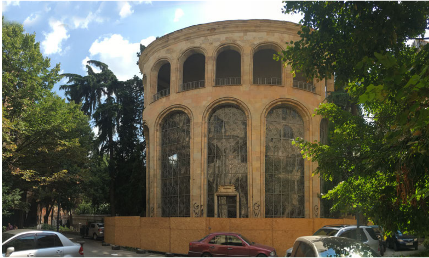
View of the exterior of the lower station building [Image: authors]
