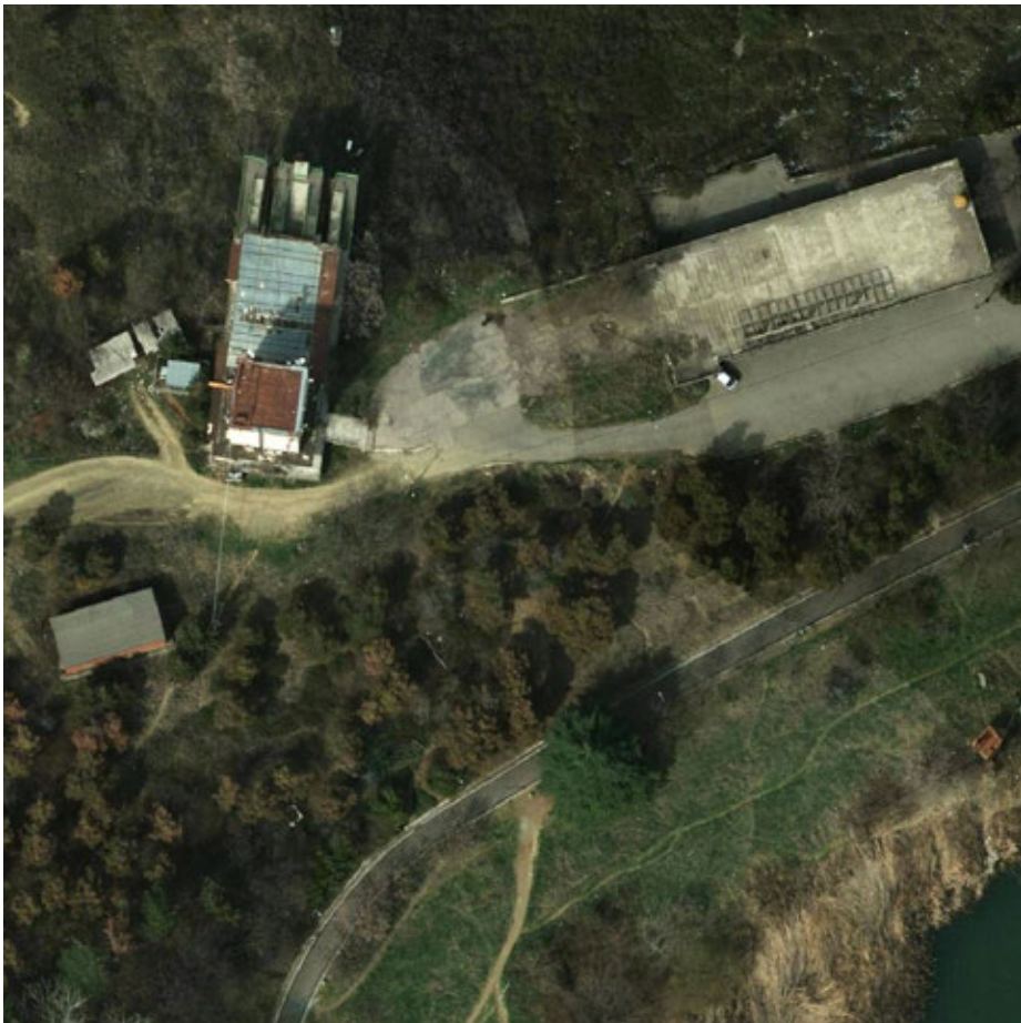
Aerial view of the upper station building
