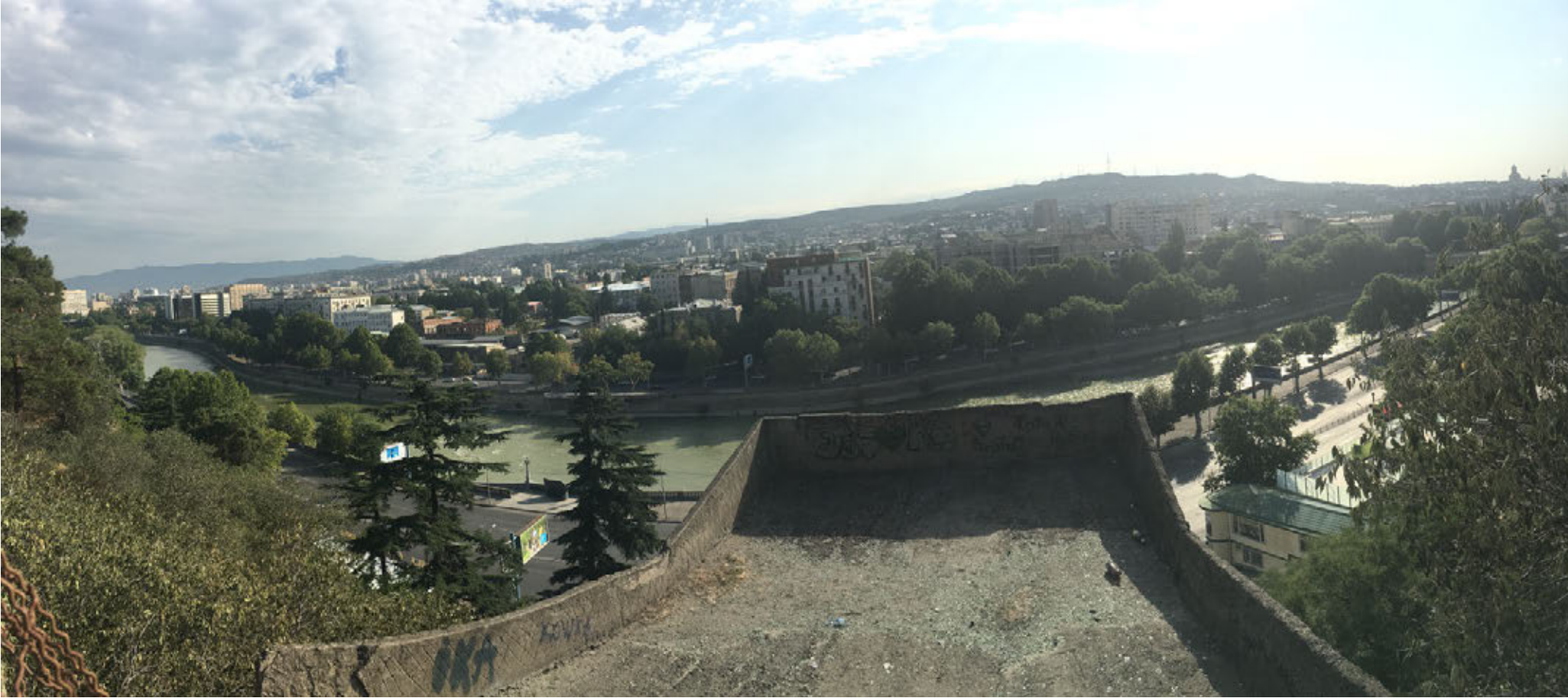
Panoramic view of the upper station platform inside Vera Park [Image: authors]
