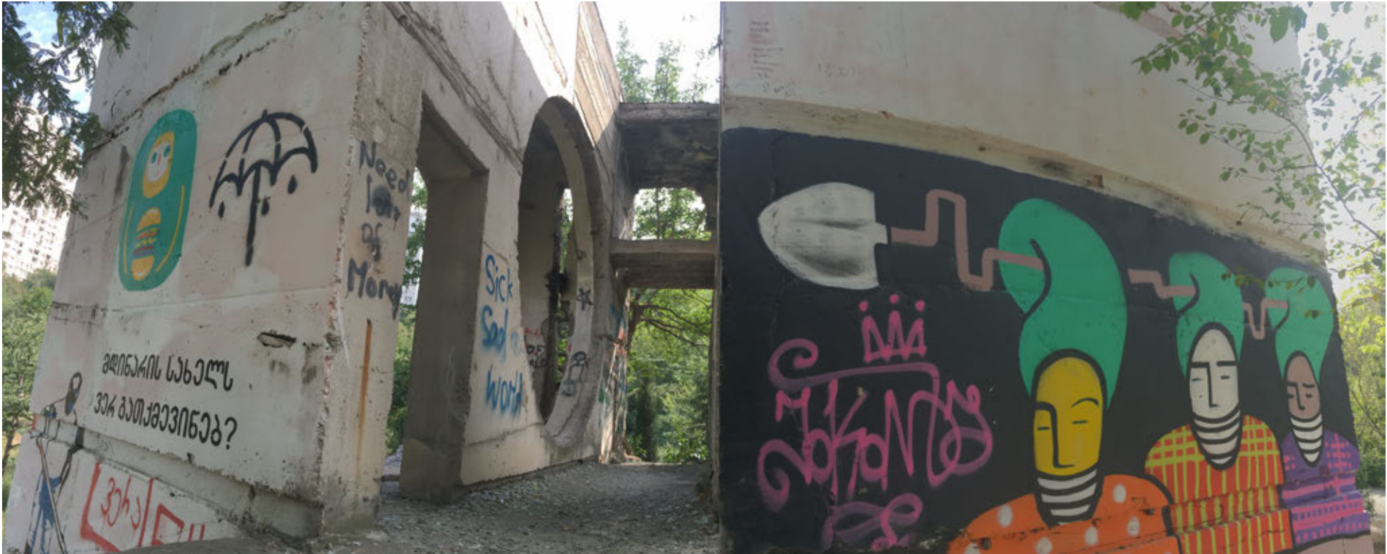
Panoramic view of the interior of the lower station building inside Mziuri Park
