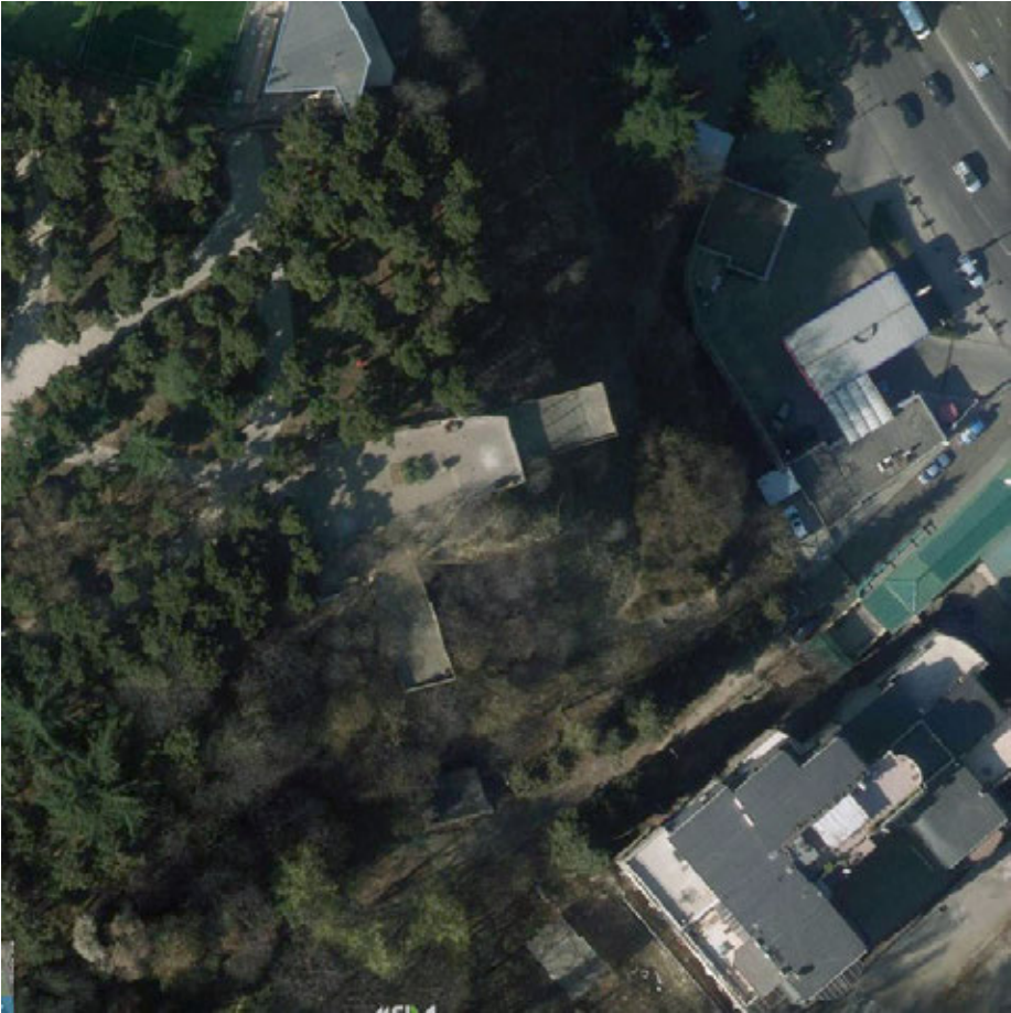
Aerial view of the upper station platform inside Vera Park
