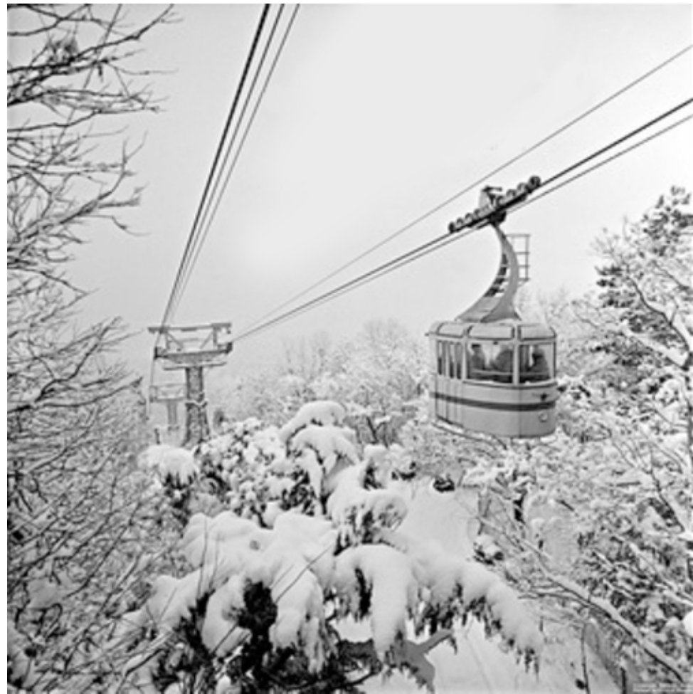
View of the cable car line in contex with the city, 1977 [Image: Malkhaz Datikashvili]
