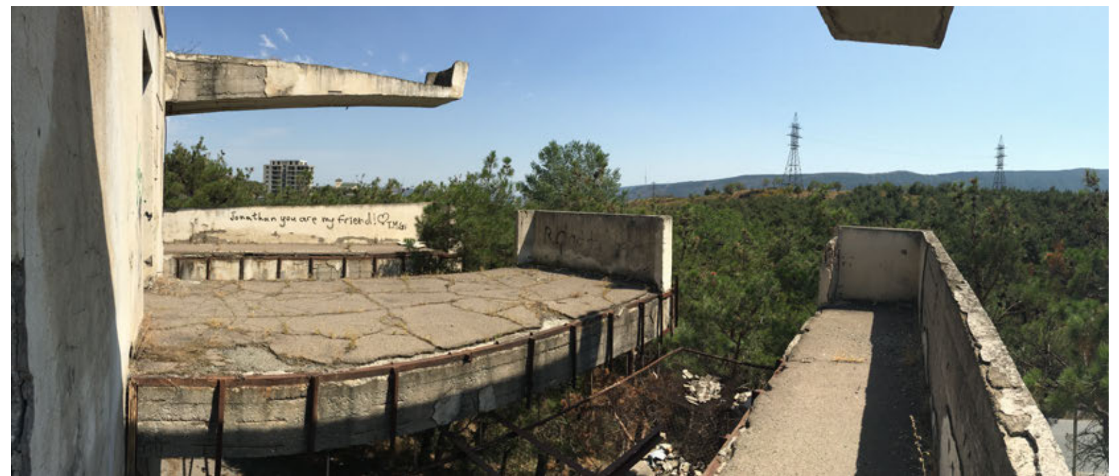
View of the of the upper station platforms [Image: authors]
