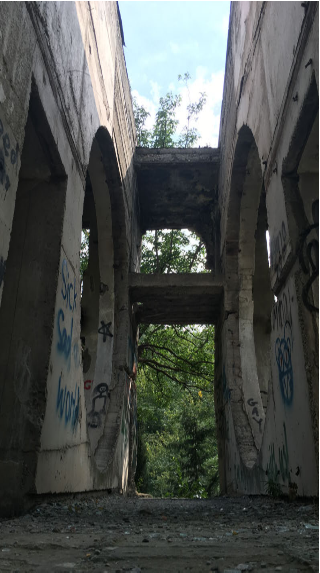
View of the interior of the lower station building inside Mziuri Park
