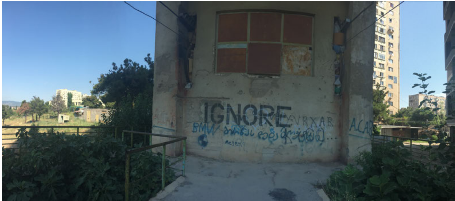
View of the exterior of the upper station building, with graffiti by Sadarismelia [Image: authors]
