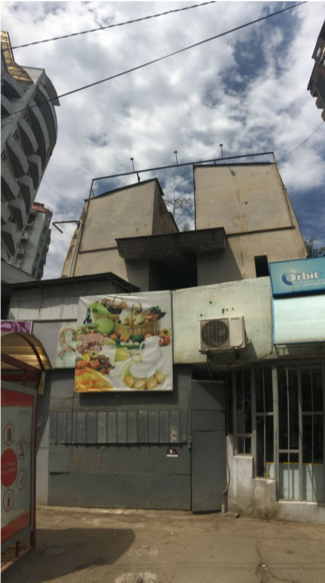
View of the of the lower station building [Image: authors]
