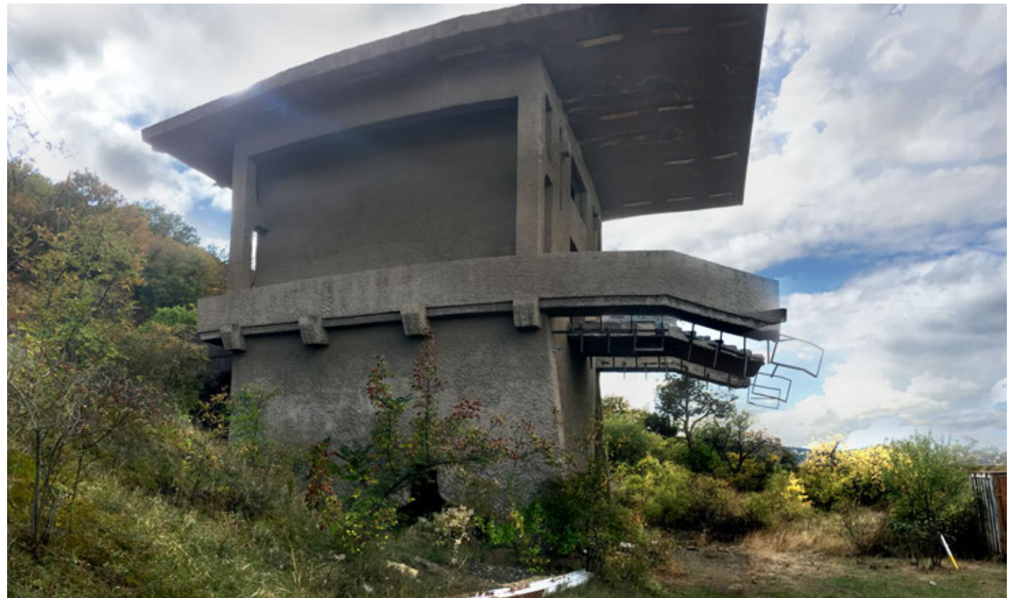
View of the platforms of the upper station building [Image: authors]
